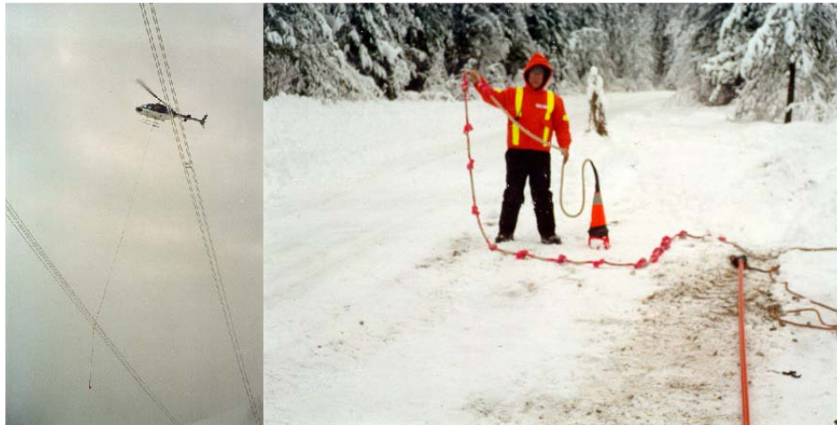
Figure 7.12: Helicopter use of 90-kg weight with large knotted rope
