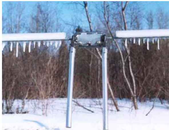
Figure 7.11: Twisting device installed at mid-span of a ground wire [96]
