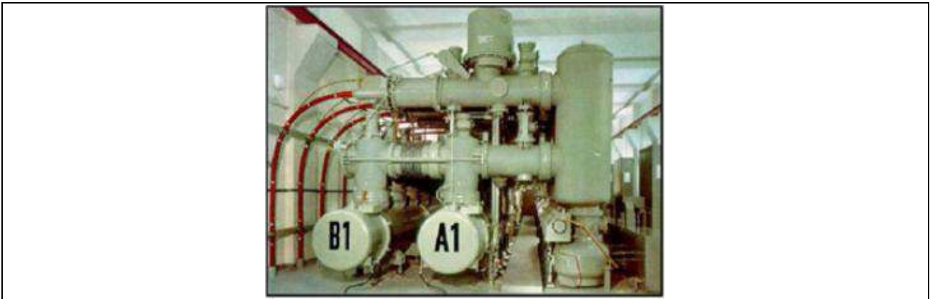
Figure 8: "UW Wittenau", one of the first SF 6 GIS ever manufactured
