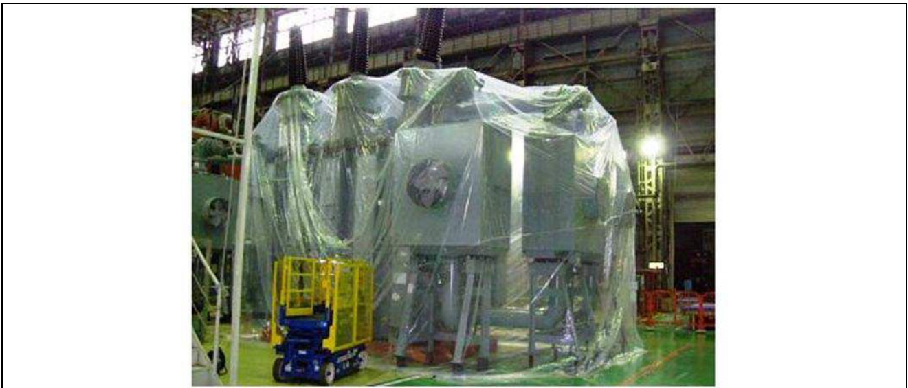
Figure 13: Leakage test on 39 MVA – 132 kV / 11 kV GIT
