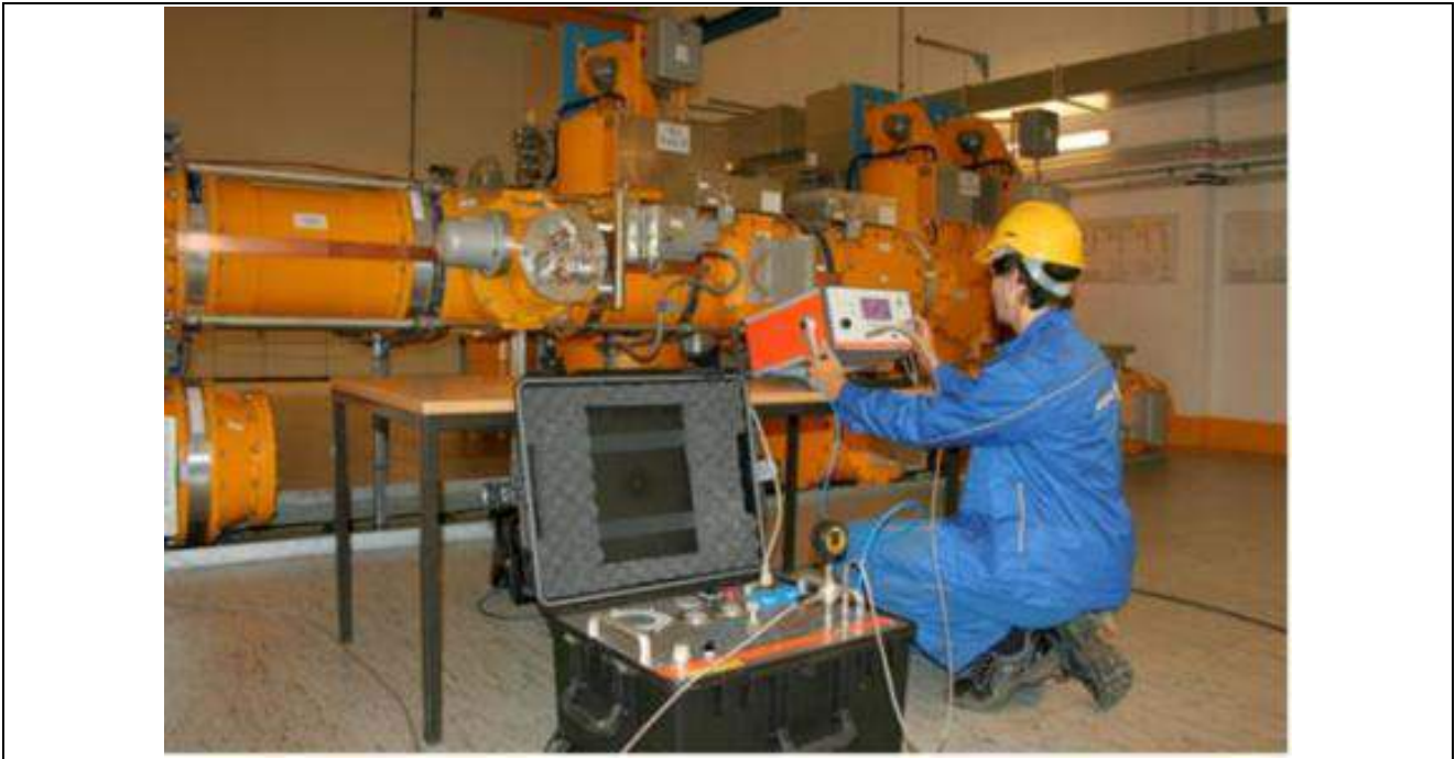
Figure 9: SF 6 collecting device in service
