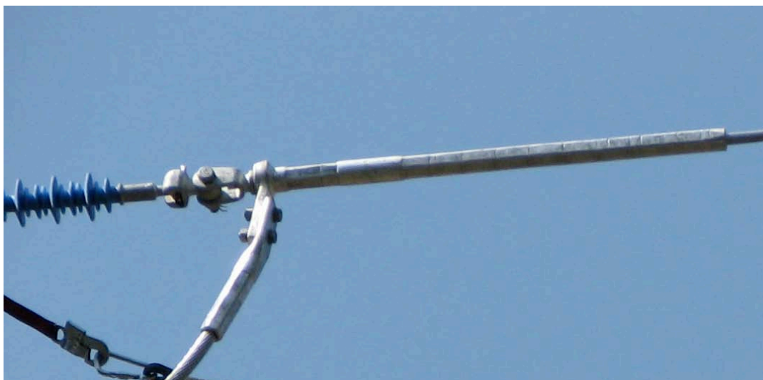
Figure 41: Hexagonal die compression clamp.
