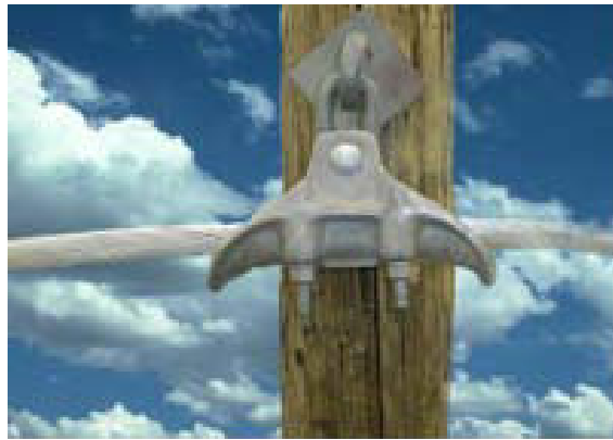
Figure 19: Typical bolted suspension clamp on bare conductor.
