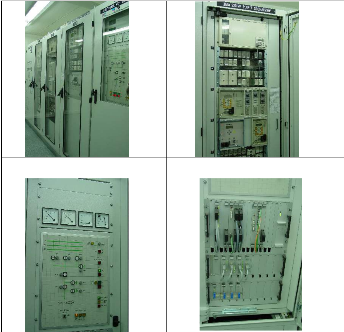
Figure 7. Protection and Control cubicles layout
