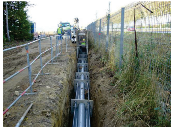
Installation in ducts
