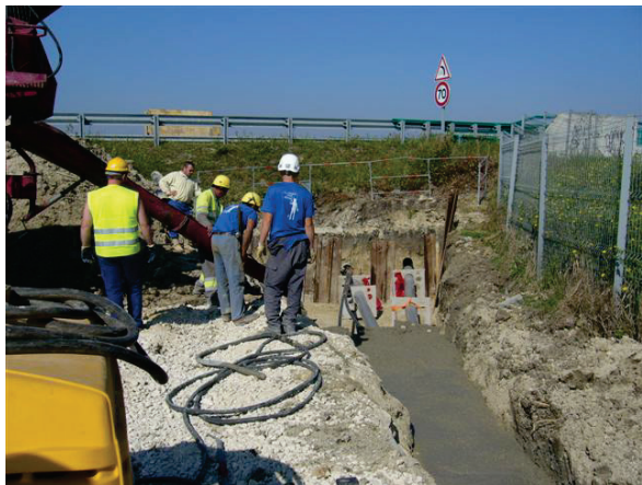
Pulling of the cables
