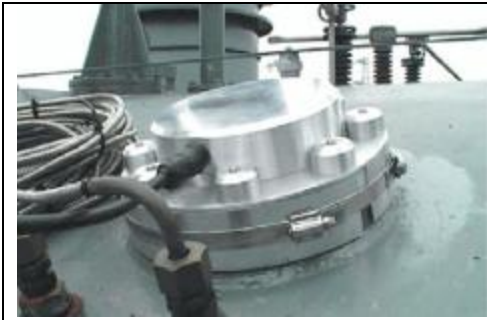
Fig. 3.2: Externally mounted UHF sensor on the tank of a 1000 MVA transformer [13]
