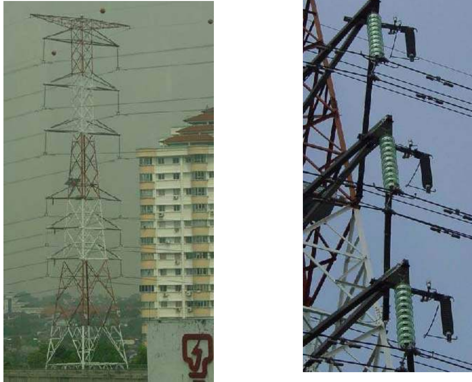
Figure 22 Quadruple circuit transmission line with line surge arresters installed on the 132 kV circuit.
