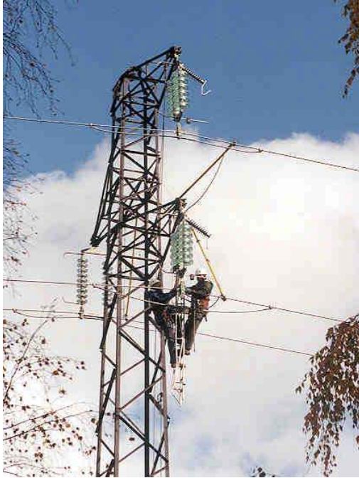
Figure 2: Left picture: RTE employees (France) installing line surge arresters on a 90 kV tower (extracted from [20]); Right Picture: Line surge arresters are installed on a high alpine 110 kV line by a KELAG service team (courtesy KELAG, Austria).
