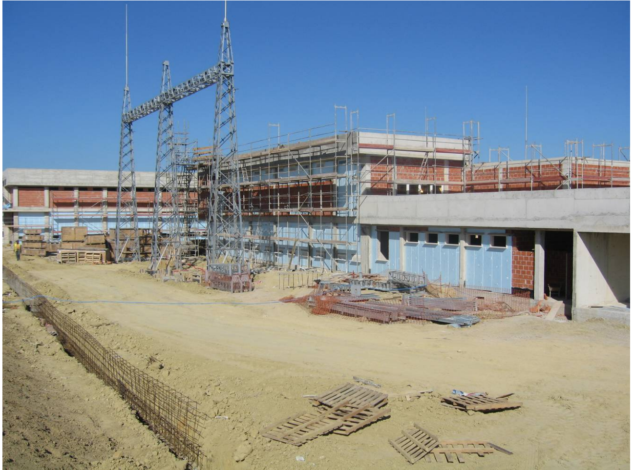
Construction phase of the substation main buildings
