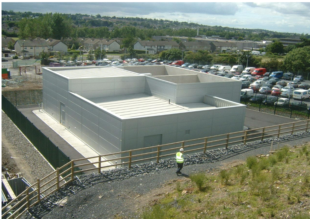
Fig 3. Typical 110kV/MV GIS Substation – After Completion
