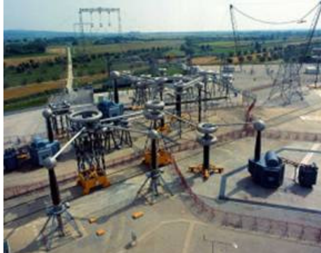
Figure 7.1.2 Italian Suvereto UHV testing station
