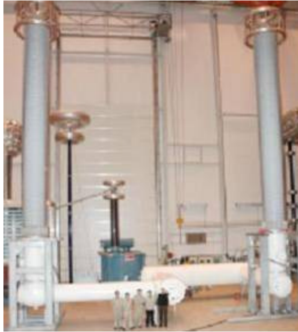
Figure 7.6.2 Test pole for bus-charging switching tests [11]
