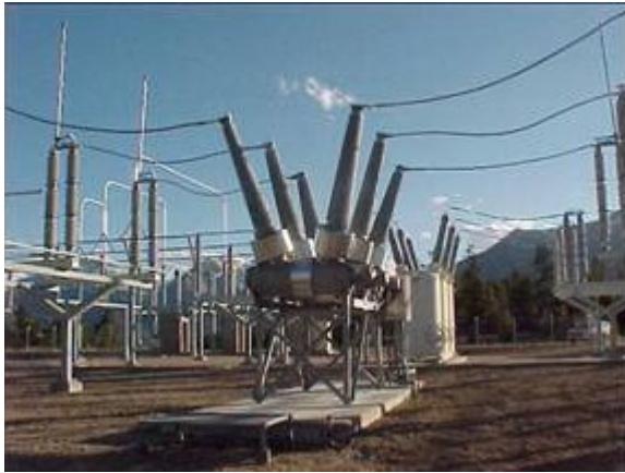
a) Composites on dead tank circuit-breaker
