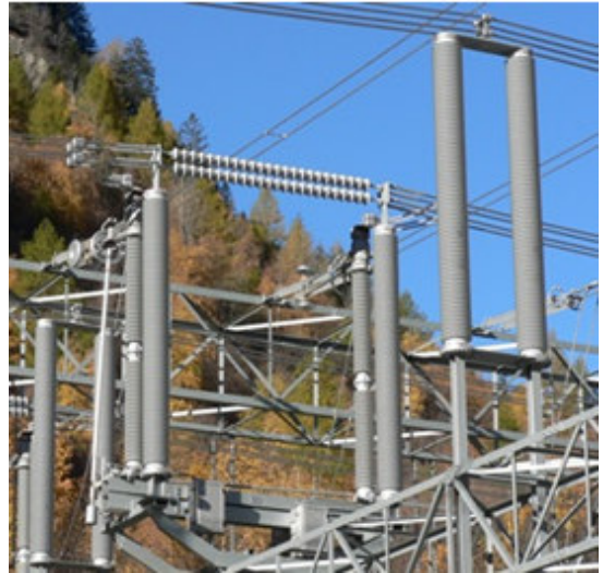
b) 420 kV AC station post insulator
