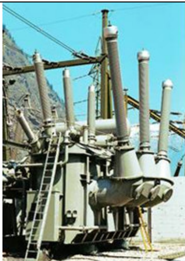
Figure 2-4: Composite bushing for HV power transformer
