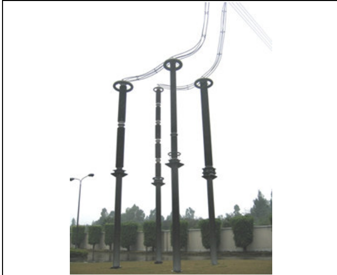
a) 500 kV DC station post insulator
