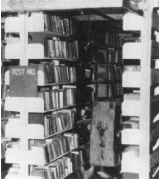
FIGURE L.1(i) Close-up of Extent of Fire Damage After Test 1 with Automatic Sprinklers. (Note limited area of fire damage.)
