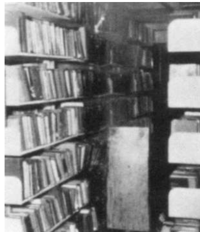
FIGURE L.1(h) After Fire Extinguishment by Sprinklers; Fire Damage to Books in Only 10 Percent of Space.
