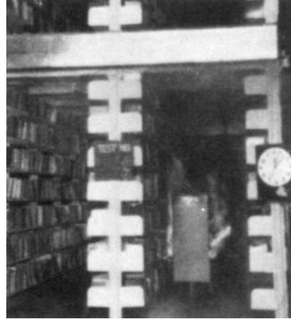
FIGURE L.1(g) Eight Minutes, 3 Seconds; Two Sprinklers Operating; Fire in Stack Under Control.
