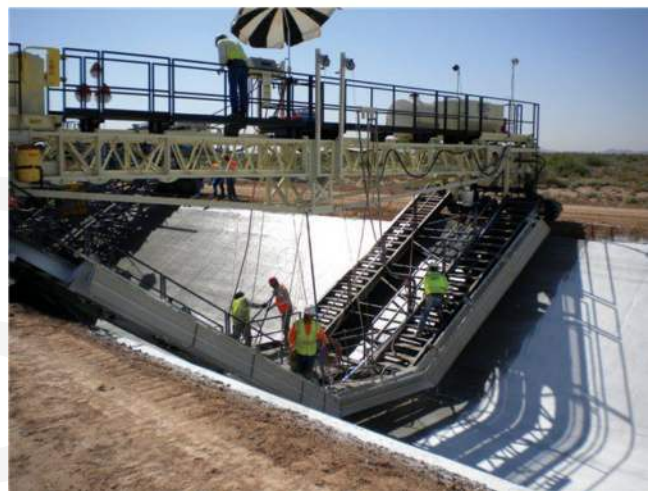
Fig. 5.1c—Concrete canal reinforced with steel mesh (top) and 7.5 lb/yd 3 (4.5 kg/m 3 ) of synthetic macrofiber (bottom) (Pima-Maricopa Irrigation Project, Sacaton, AZ).
