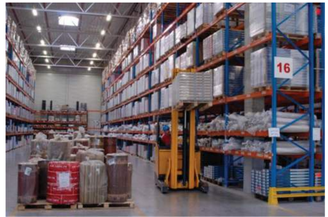
Fig. 5.2a—FRC warehouse using high-aspect-ratio steel fibers at a dosage of 51 lb/yd 3 (30 kg/m 3 ) with extended joint spacing (Stykov, Poland).
