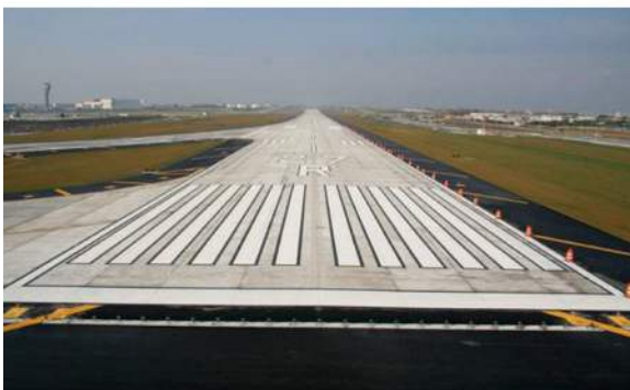
Fig. 5.1b—Concrete runway reinforced with 66 to 85 lb/yd 3 (39 to 50 kg/m 3 ) of steel fibers (O'Hare Airport runway, Chicago, IL).
