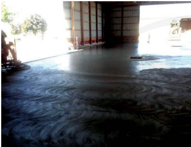
Fig. 5.2c—FRC warehouse with extended joint spacing using synthetic macrofibers at 7.5 lb/yd 3 (4.5 kg/m 3 ) and low-shrinkage concrete (Champaign, IL).
