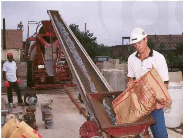
Fig. 6.3—Synthetic and steel macrofibers being added to the mixer truck.
