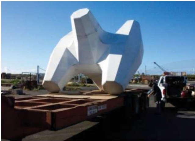
Fig. 5.5b—Precast Pi section made with ultra-high-performance steel FRC (Jackway Park Bridge, IA).
