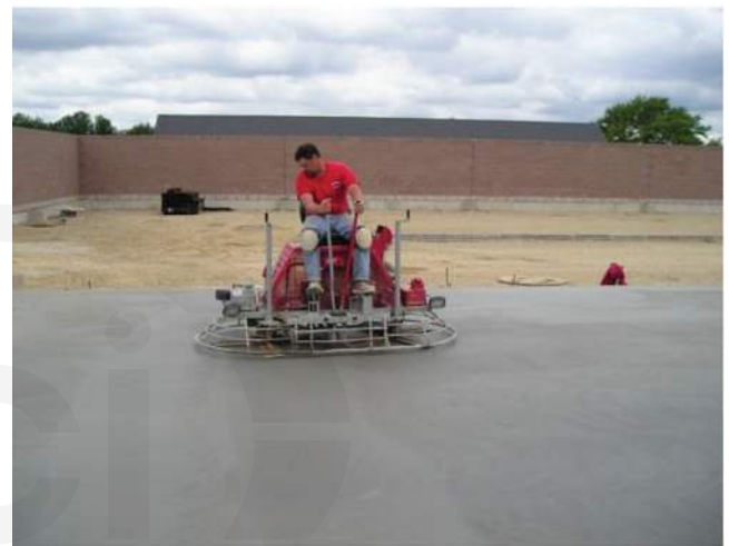
Fig. 6.4—FRC can be finished with similar tools used for unreinforced concrete.
