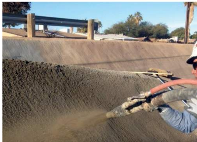
Fig. 5.6a—Canal repair using synthetic macrofiber shotcrete in Phoenix, AZ.
