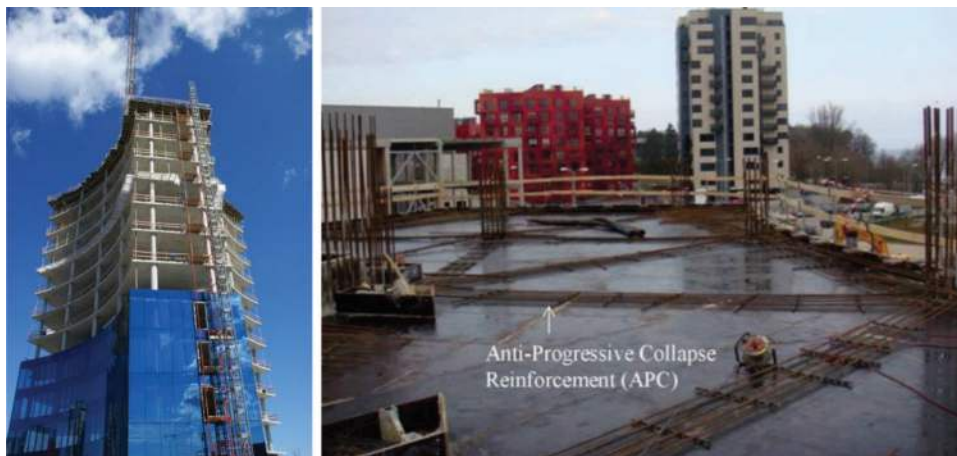
Fig. 5.3—Construction of a multi-story building with SFRC elevated slabs. Note that the only bars in the suspended slabs are between columns as anti-progressive collapse reinforcement and the slab itself is reinforced with steel fibers only ( ACI 544.6R ).
