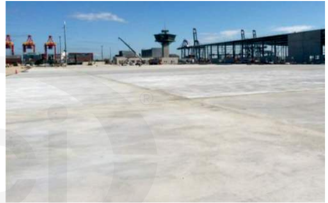
Fig. 5.2b—Seamless 538,000 ft 2 (50,000 m 2 ) FRC pavement using high-aspect-ratio steel fibers at a dosage of 42 lb/yd 3 (25 kg/m 3 ) plus wire mesh (Port of Brisbane, Australia).
