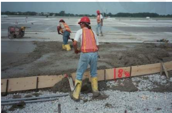
Fig. 5.1a—Concrete slab-on-ground reinforced with 4.3 lb/yd 3 (2.5 kg/m 3 ) of synthetic macrofiber (Cleveland Medical Mart and Convention Center, Cleveland, OH).
