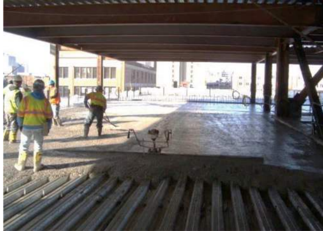
Fig. 5.4—Concrete slab on metal deck reinforced with 4 lb/yd 3 (2.4 kN/m 3 ) synthetic macrofibers (22-story steel frame building, Newark, NJ).
