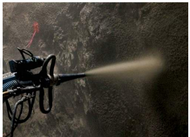
Fig. 5.6b—Rock stabilization using steel fiber-reinforced shotcrete.
