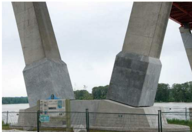
Fig. 6.3—(a) Seismic reinforcing bar splice retrofit (Massicotte et al. 2013); (b) casting of Mission Bridge UHPC jacket (Kennedy et al. 2015); and (c) final Mission Bridge UHPC jackets (Kennedy et al. 2015).
