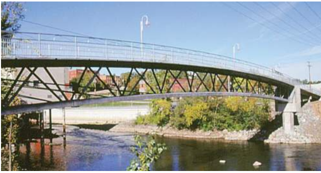
Fig. 6.2a—Sherbrooke Pedestrian Bridge (photo courtesy of Lafarge).
