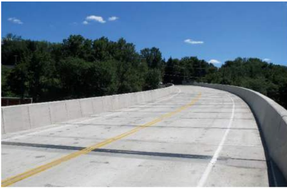
Bridge with UHPC connections
