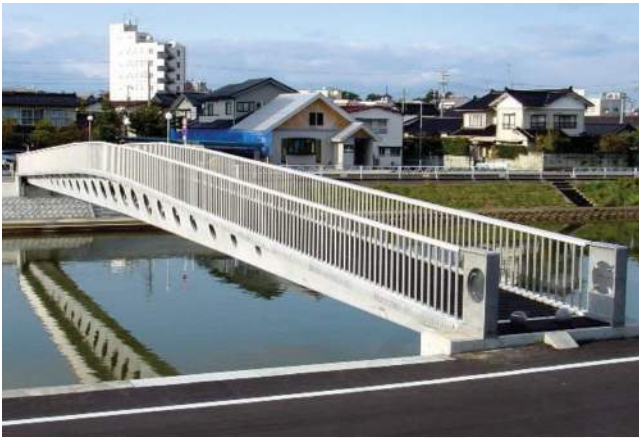
Fig. 6.2b—Sakata-Mirai Bridge (photo courtesy of Lafarge).
