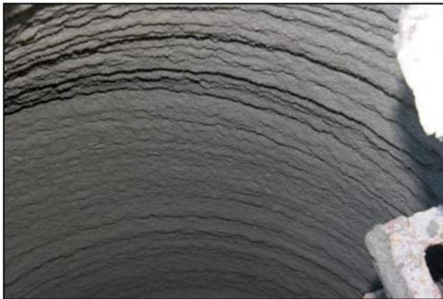
Fig. 6.11b—Rotating spray nozzle and finished sprayed surface (photos courtesy of City of Naperville).
