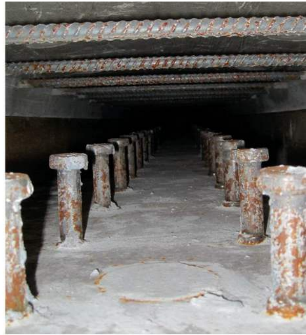
Composite connection detail
