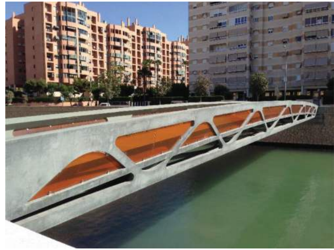
Fig. 6.2d—Pedestrian Bridge over Oveja's ravine, Alicante, Spain (photo courtesy of B. Massicotte).
