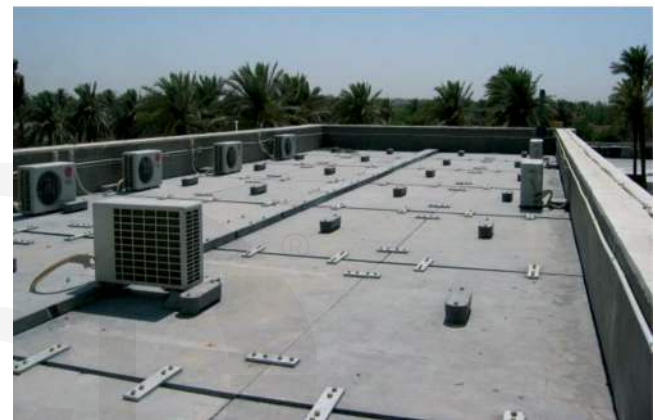
Fig. 6.7c—UHPC roof security panels ready for delivery and after installation (Cavill et al. 2006).
