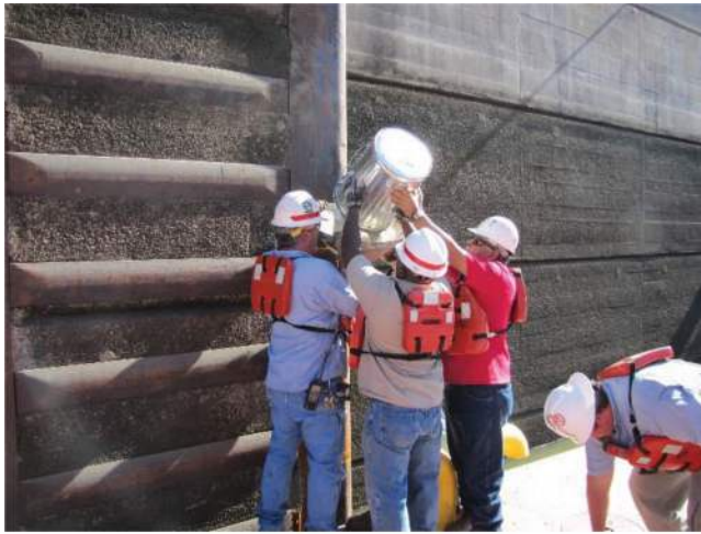
(a) Placement of repair material by pouring through ports (photo courtesy of Robert Moster)
