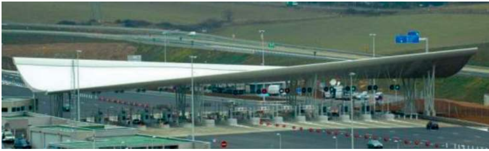
Fig. 6.12b—General overview of Millau Viaduct toll gate roof.
