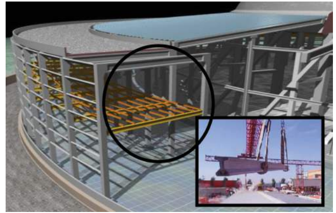
Fig. 6.11d—UHPC beams for Cattenom Nuclear Cooling Tower (Toutlemonde et al. 2009).
