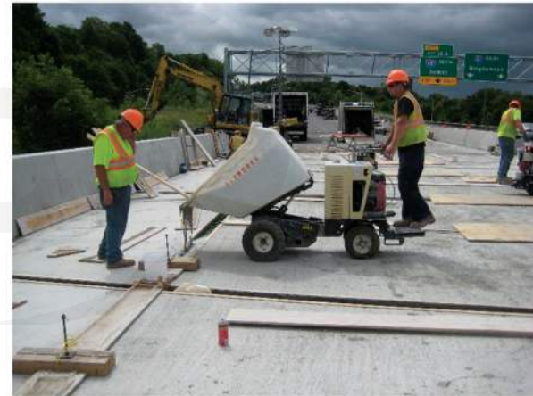
Field casting of UHPC
